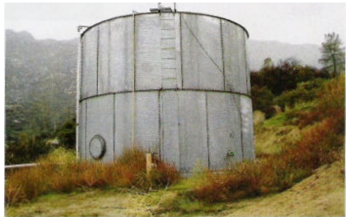
40,000-Gallon Storage Tank at Lower Site
